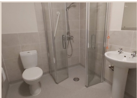
Typical shower room
