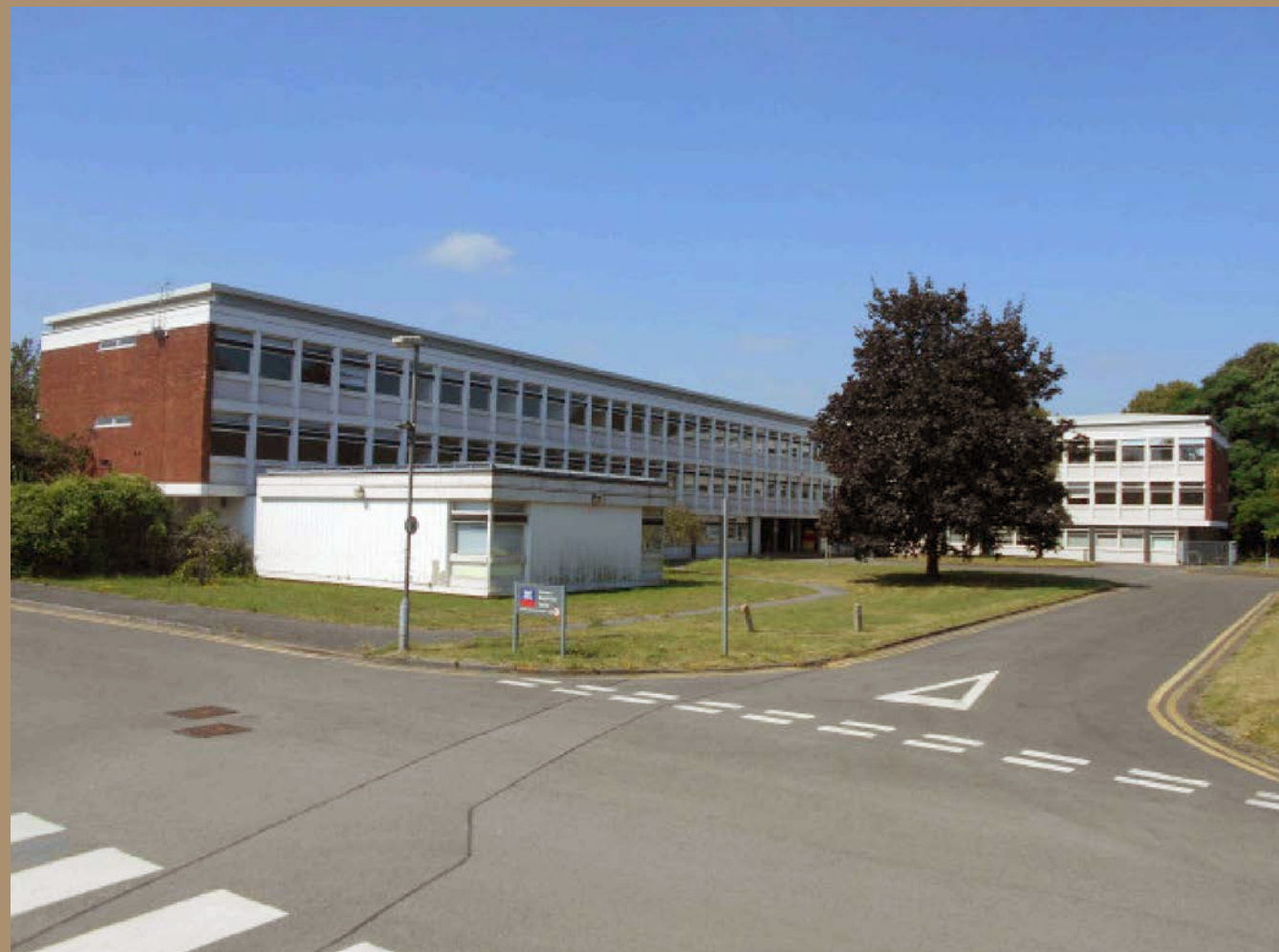
Former DEFRA Building on the Site (Demolished)
