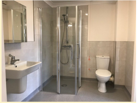
Typical shower room
